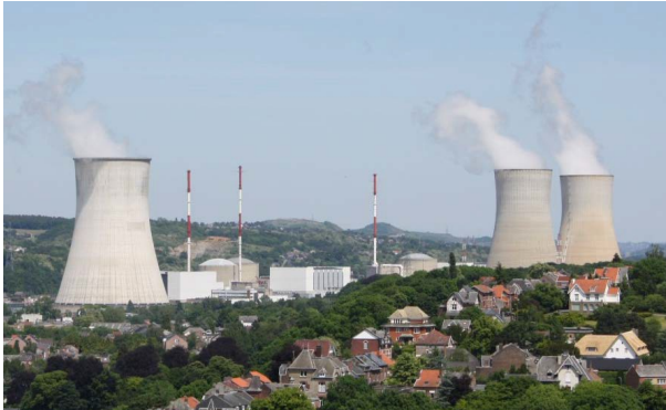
Figure 44: A nuclear power plant in Belgium. This produces nearly 3000 MW (megawatts) of power. It has 3 nuclear reactors (in the domed buildings) and 3 cooling towers
